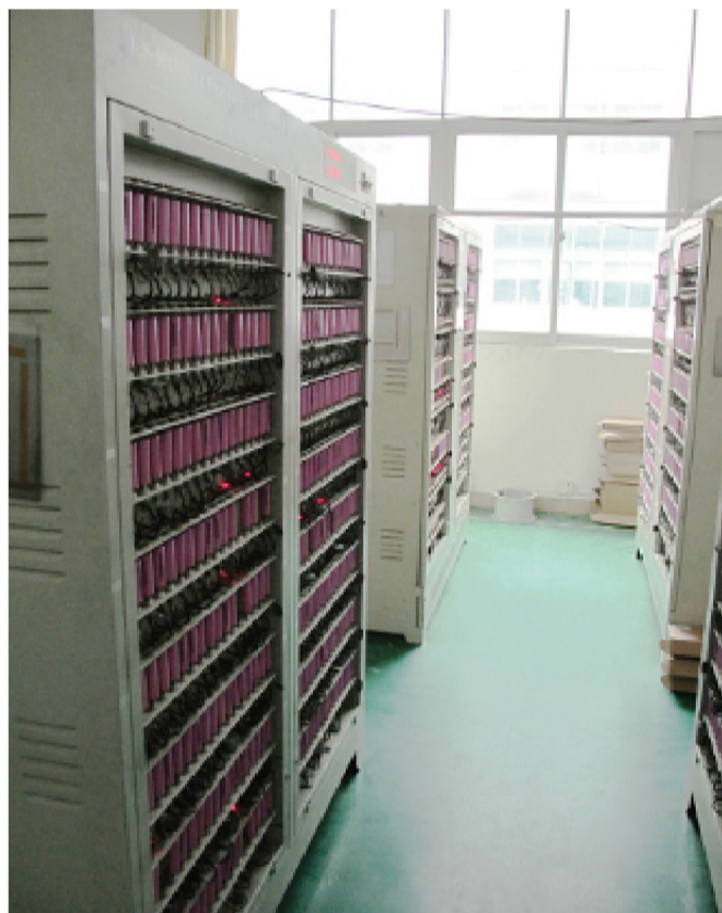
8 LUXA2 batteries under going battery-burning test
